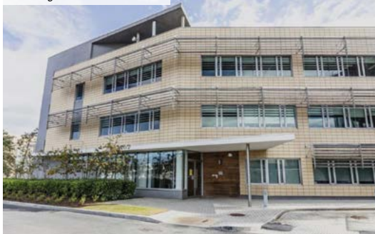
Building 8 – Dublin – Irlande
